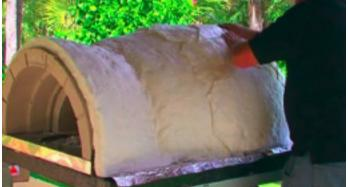
Start at the front, finish at the back ensuring complete coverage. Excess insulation must be used to plug gaps. Cut a hole for the flue.
