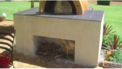
The concrete slab (top of base) must be dry, level and clean before commencing oven construction. A concrete sealant is recommended to prevent the oven drawing moisture from the base.
