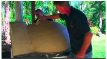
Insert the flue into the front chamber hole with the seam of the flue facing the back of the oven before beginning the rendering process. Use a spirit level to ensure the flue remains straight. For best results, use a steel float to apply the render mix.
